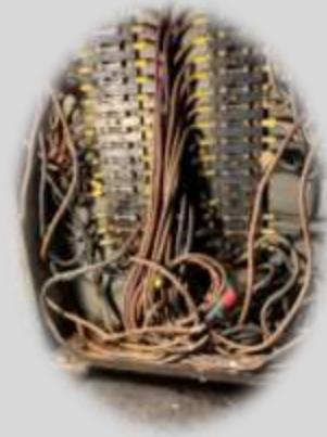
$75,000-Electrical system upgrades
