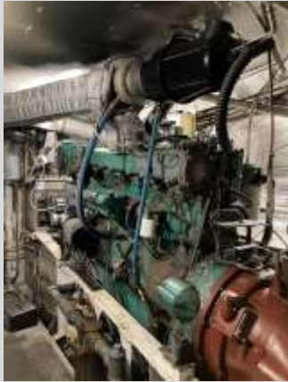
$250,000-New engines to replace original 1968 Cummins engines
